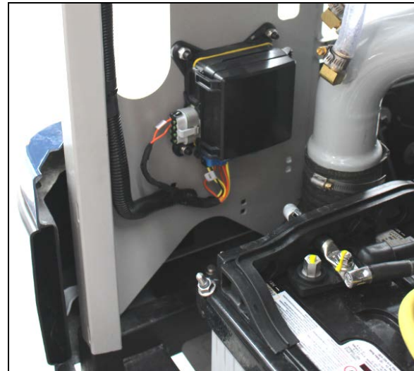
FIGURE 45: VECT (COTE TROTTOIR)
