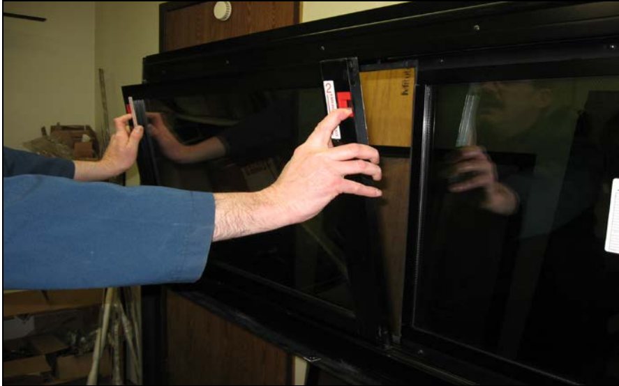
FIGURE 100: REMOVING THE SASH
