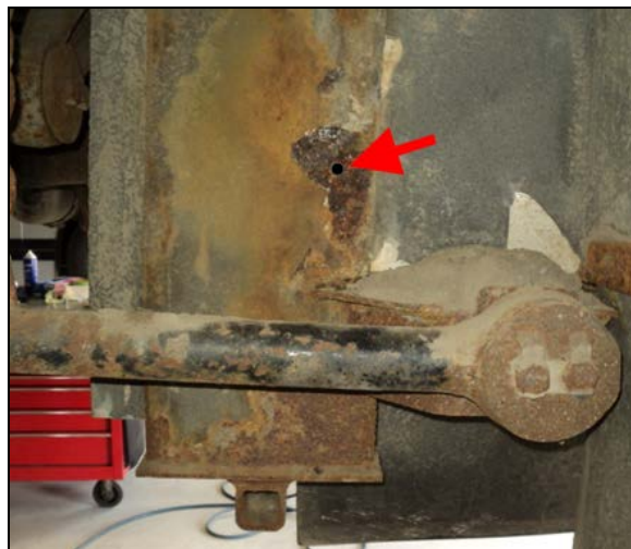
FIGURE 7: HOLE DRILLED IN STRUCTURAL MEMBER
