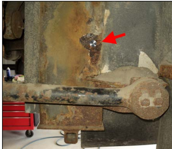
FIGURE 6: CLEANED SPOT ON STRUCTURAL MEMBER
