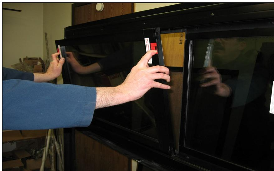
FIGURE 103: RETRAIT DU CHÂSSIS
