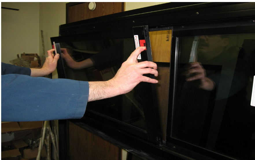
FIGURE 47: REMOVING THE SASH
