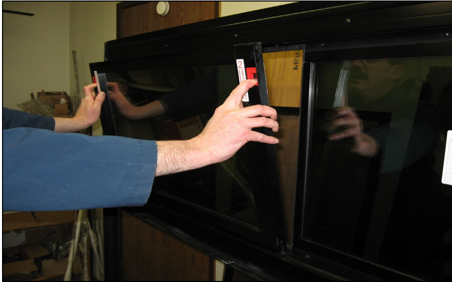
FIGURE 107: REMOVING THE SASH
