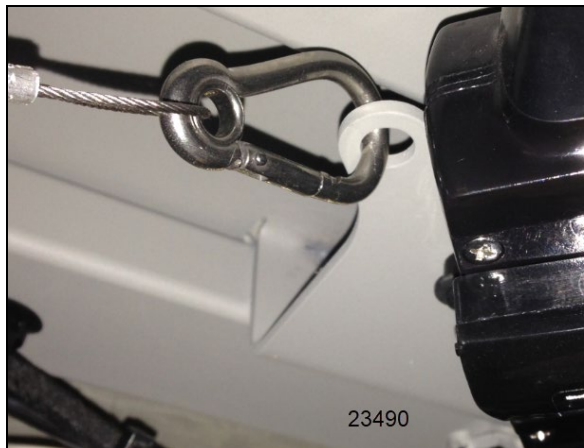
FIGURE 58: PROTECTIVE WIRE INSTALLATION
