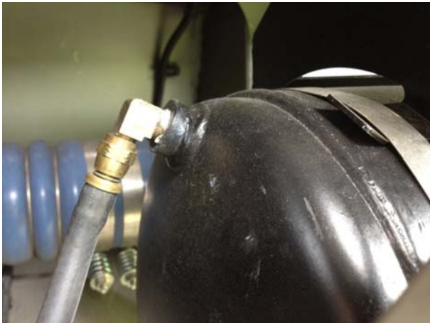
NEW COOLANT SURGE TANK INSTALLED – ROAD SIDE
