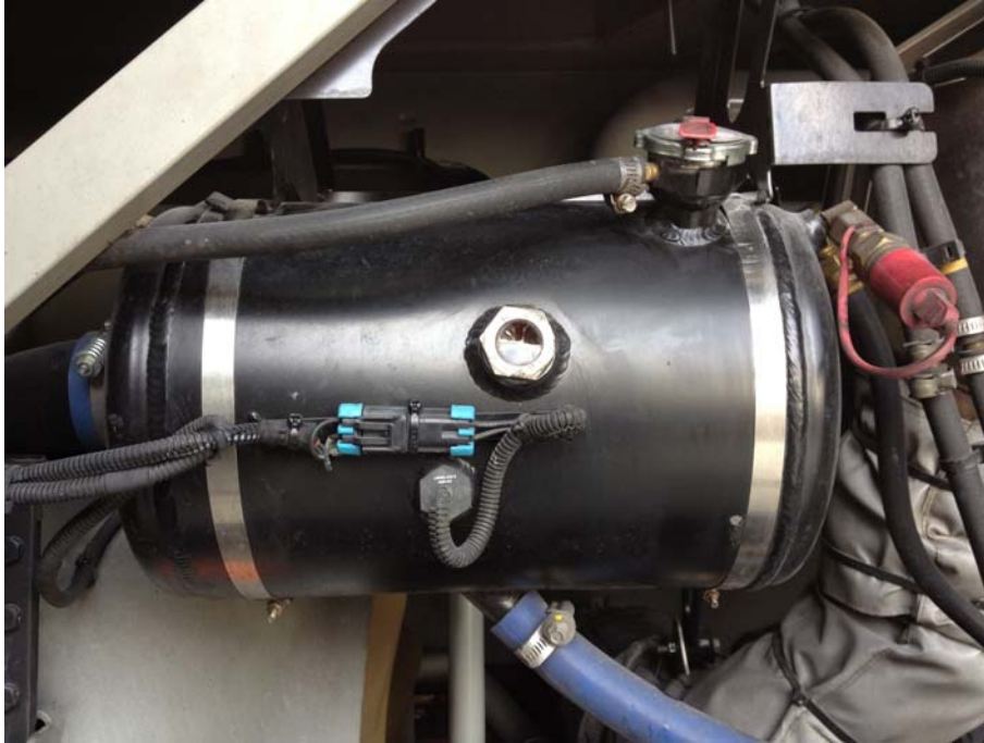
NEW COOLANT SURGE TANK INSTALLED
