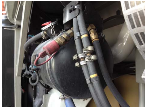
NEW COOLANT SURGE TANK INSTALLED – CURB SIDE
