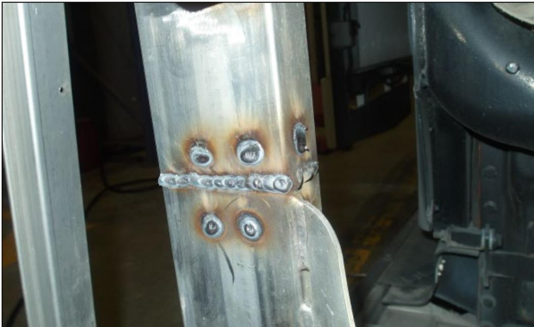
13. For aesthetic considerations, the welds must be ground off and the support sanded to a semi-smooth finish that will closely as possible match the natural beam finish.
