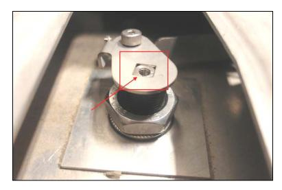
15. Secure the latch plate to the handle using the supplied screw, lock and washer (5001377, 5001137 & 5001544).
