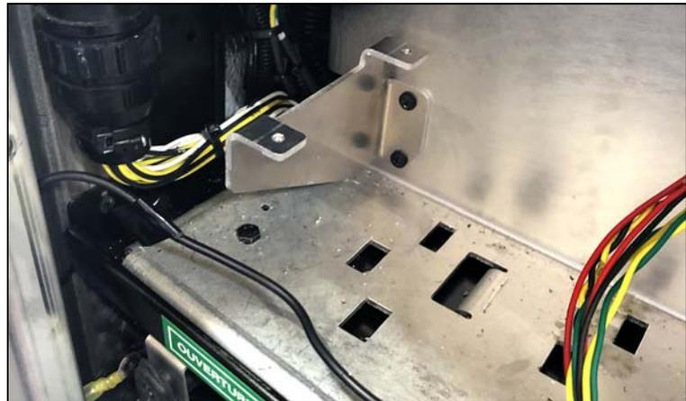
FIGURE 26: BRACKET RELOCATION.
