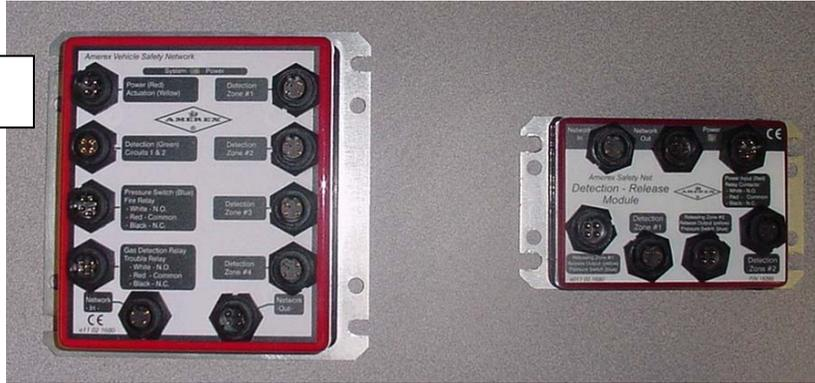
Option 3: A fire detected on either module (A or B) activates only that module, but a Manual Release button located anywhere in the system releases all Fire Suppression systems.
