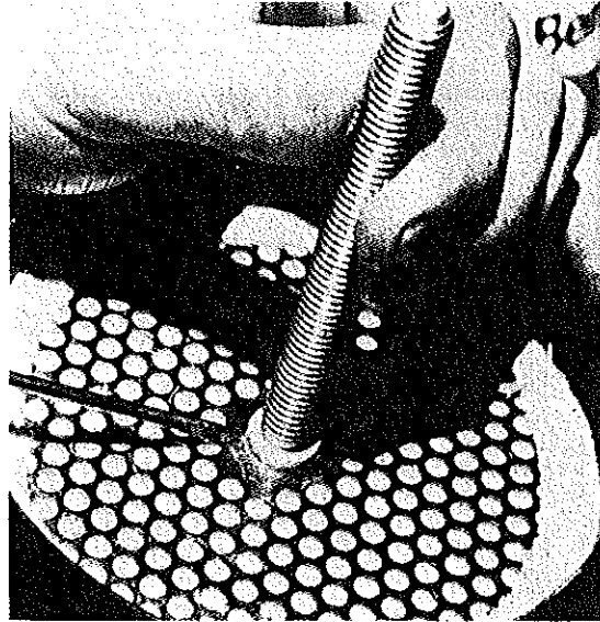
Installing perforated plate into shell
