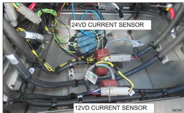
**FIGURE 11: 12VD / 24VD CURRENT SENSORS IN MPC (TYPICAL)**
