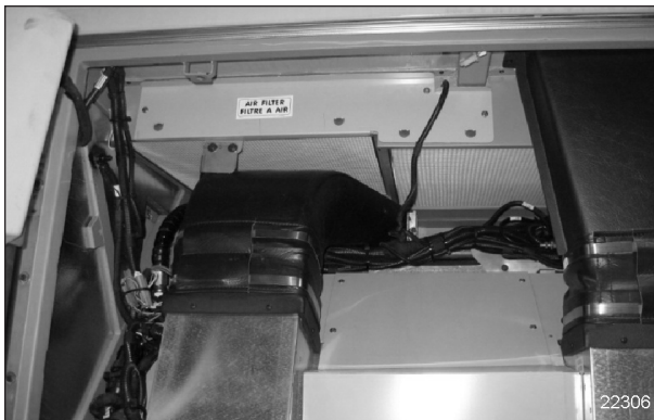
FIGURE 16: CABIN AREA AIR FILTER
