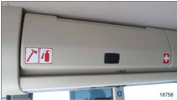
FIGURE 10: A DECAL INDICATES THAT A FIRE HATCHET, A FIRE EXTINGUISHER AND A FIRST-AID KIT ARE LOCATED IN THIS OVERHEAD COMPARTMENT
