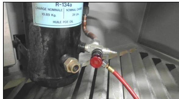
FIGURE 100: RECOVERY UNIT CONNECTED TO RECEIVER SERVICE PORT
