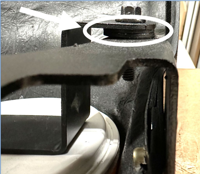
Figure 16: Two washers per screw
