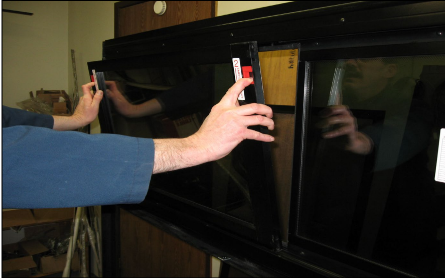
FIGURE 107: REMOVING THE SASH
