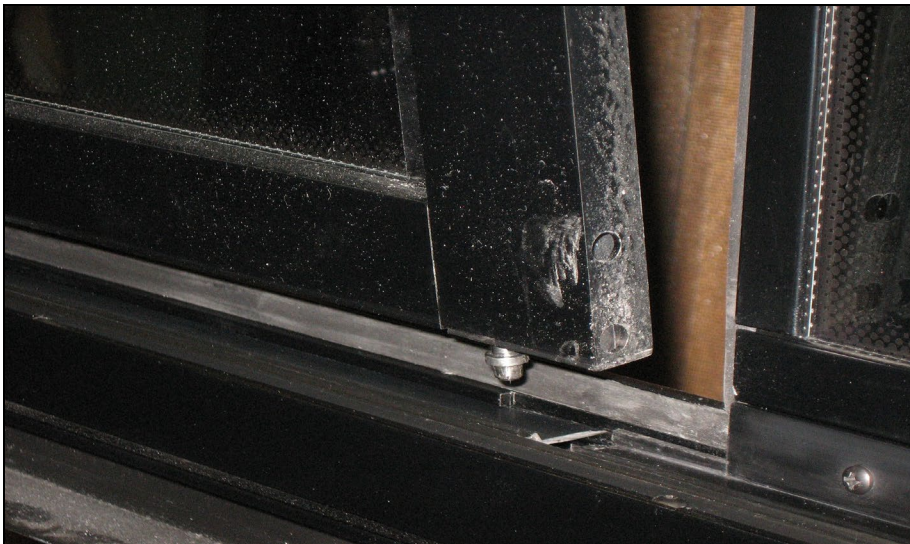
FIGURE 108: DISENGAGING THE BOTTOM OF THE SASH
