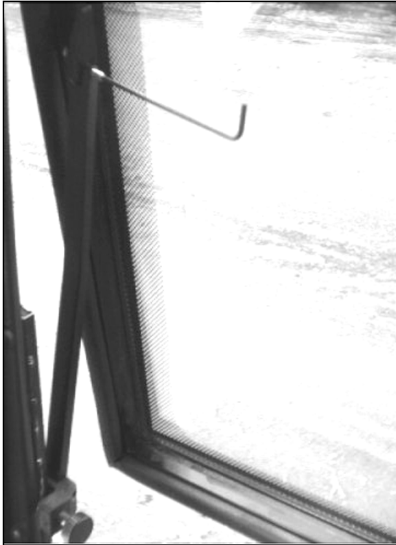
FIGURE 1: DISASSEMBLING THE STOPPER ARM FROM THE WINDOW.
