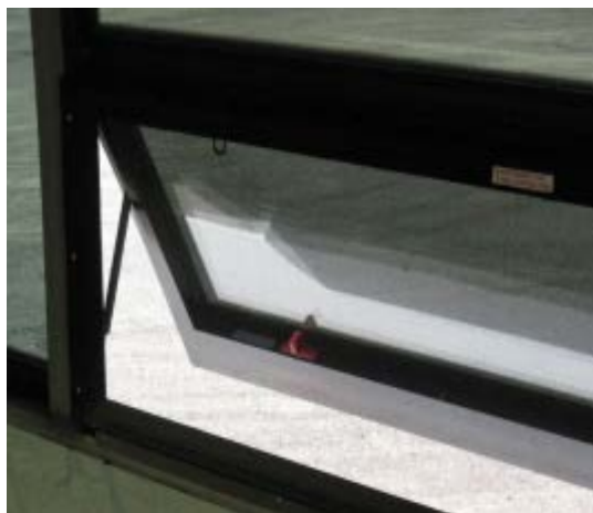
Fig.2 Inside view of an awning window
