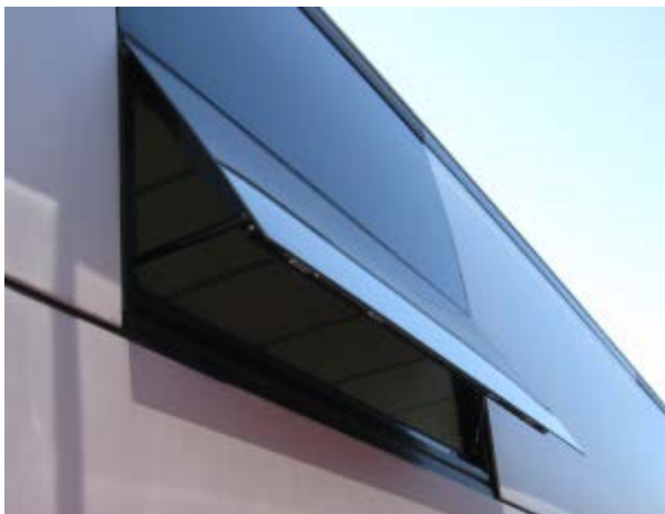
Fig.1 Typical awning-type window
