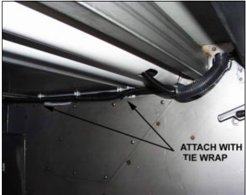
Figure 9 : attach harness and wires all along the baggage compartment ceiling
