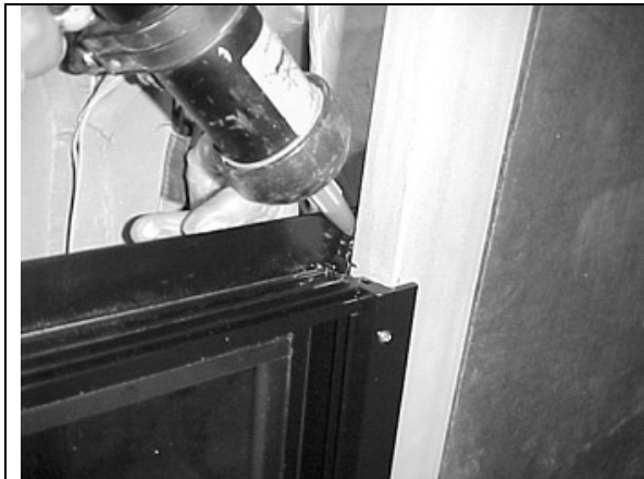
FIGURE 74 : AWNING WINDOW – SEAL THE UPPER CORNERS
