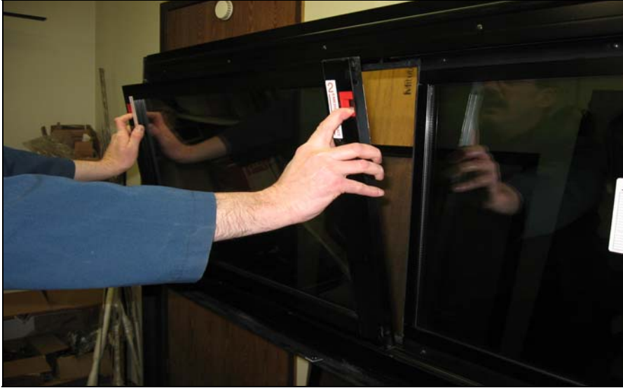
FIGURE 64: REMOVING THE SASH
