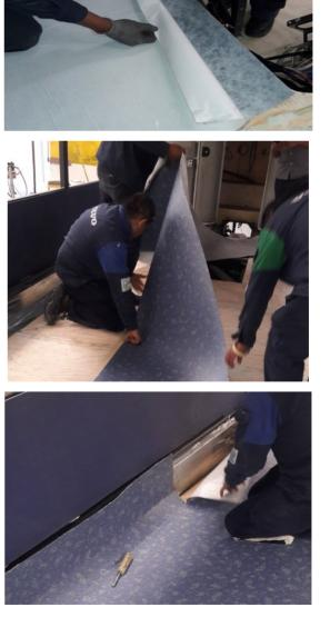
20. Press the linoleum to ensure the adhesion.
