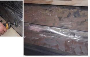
16. Sweep the wood floor so that remove dust and/or wood remains. Then use a wet cloth with thinner or alcohol to clean the plate.
