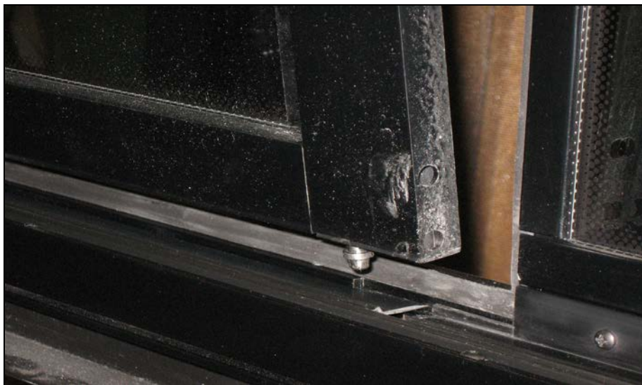
FIGURE 65: DISENGAGING THE BOTTOM OF THE SASH
