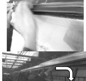
11. Start at the middle of the bottom edge of the window's frame, radius at the corners as small and smooth as possible, check the good adhesion of the rubber molding.
