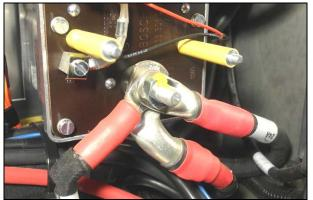
Figure 15: When several terminals are connected on a single stud terminal, the largest cable lug must be placed first, followed by the second larger and so on. Cable lugs should be distributed around the stud terminal in a way that no cable lug is distorted when tightening the nut.
