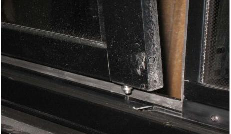
FIGURE 42: DISENGAGING THE BOTTOM OF THE SASH
