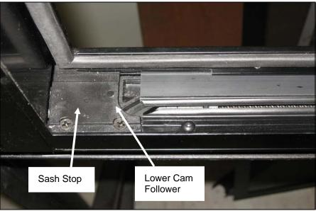
FIGURE 66: PROPER ALIGNMENT
