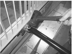
FIGURE 64: DOOR LATERAL ADJUSTMENT
