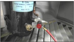
FIGURE 80: RECOVERY UNIT CONNECTED TO RECEIVER SERVICE PORT
