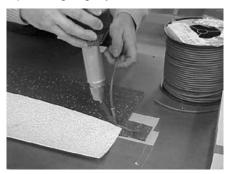
8. The heel of the fast nozzle must not lean against "Tarabus" covering (always parallel to the surface).
