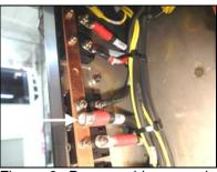
Figure 9: Power cable on main circuit breakers' bus bar.
