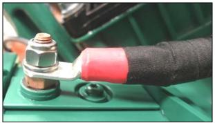
Figure 16: No exposed or broken copper strands.
