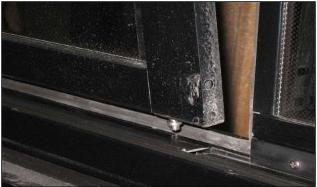
FIGURE 65: DISENGAGING THE BOTTOM OF THE SASH
