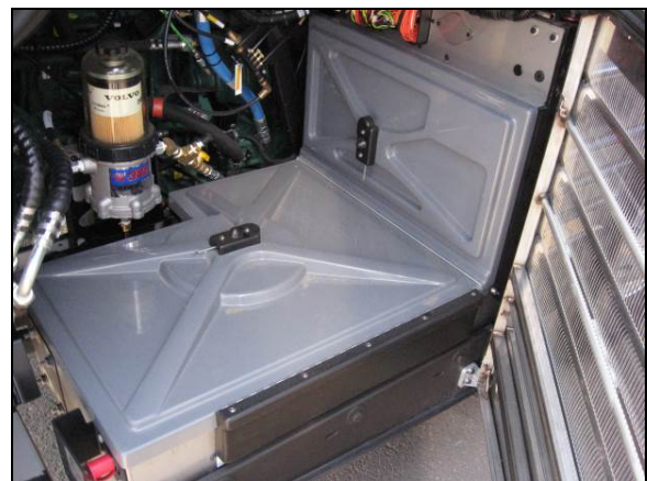
FIGURE 8: REAR ELECTRICAL PANEL, JUNCTION PANEL & BATTERY COMPARTMENT
