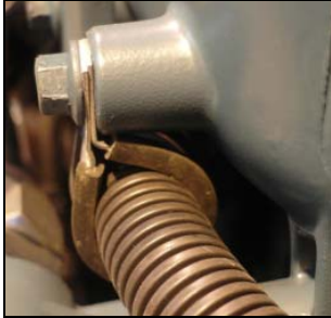
Figure 19: P-clamp with appropriate diameter prevents the power cable or corrugated protective sheath from moving and rubbing inside the clamp.
