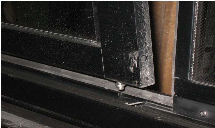
FIGURE 42: DISENGAGING THE BOTTOM OF THE SASH
