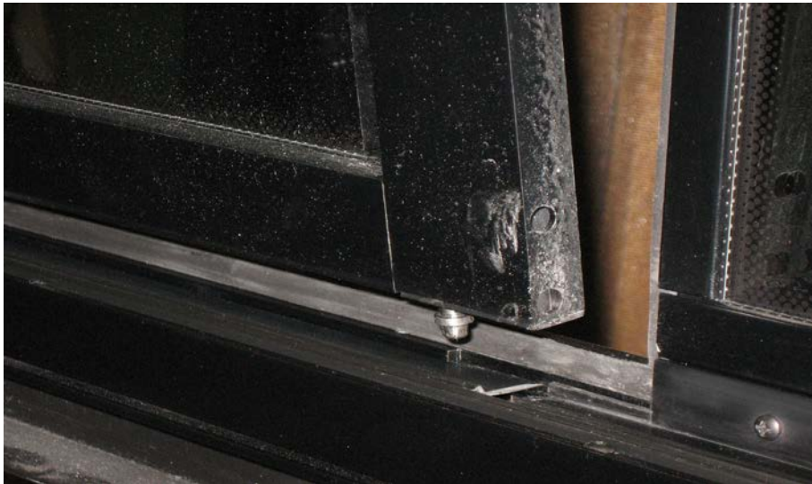
FIGURE 42: DISENGAGING THE BOTTOM OF THE SASH
