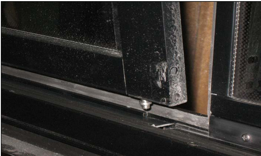
FIGURE 101: DISENGAGING THE BOTTOM OF THE SASH
