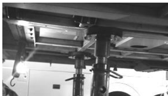
FIGURE 21: JACK STANDS UNDER THE FUEL TANK CRADLE
