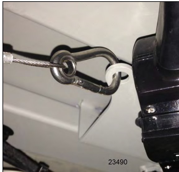
FIGURE 54: PROTECTIVE WIRE INSTALLATION
