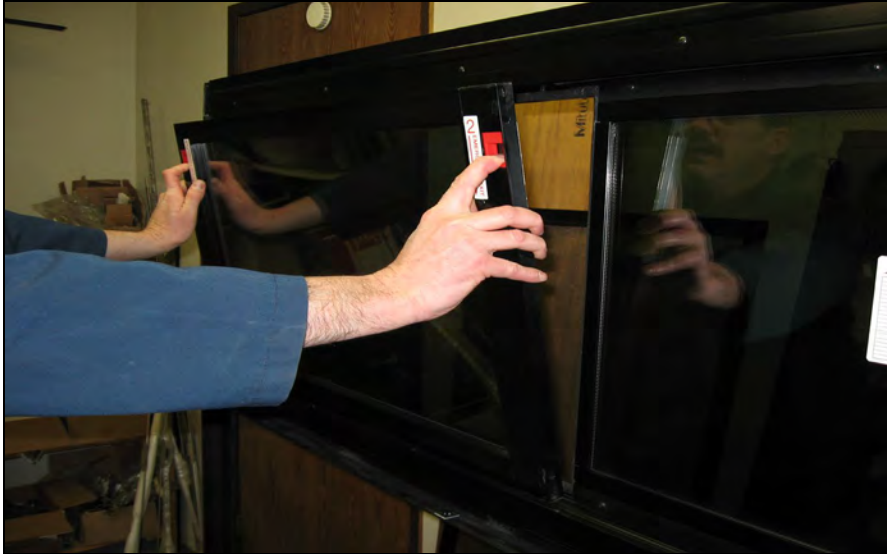
FIGURE 107: REMOVING THE SASH
