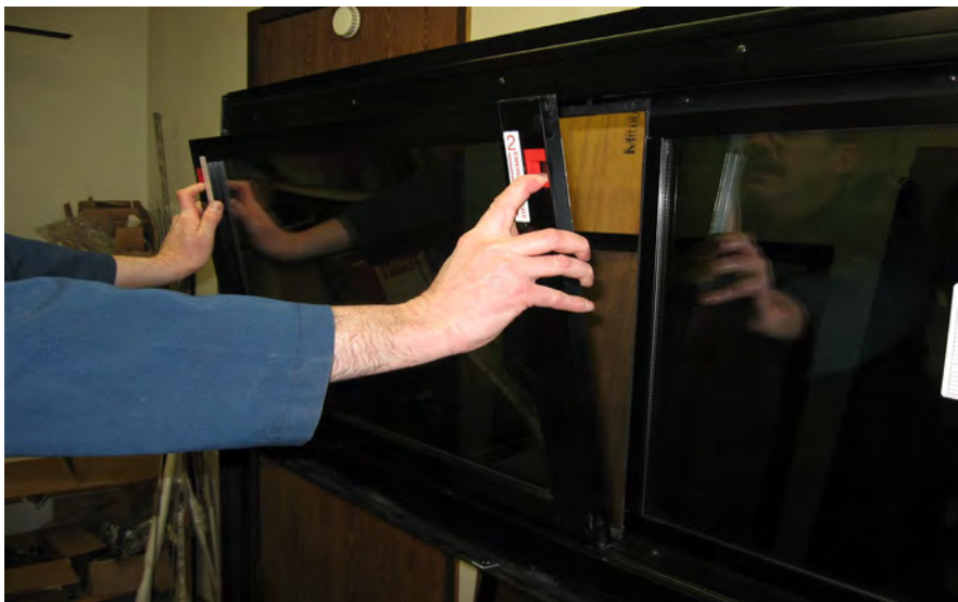
FIGURE 44: REMOVING THE SASH
