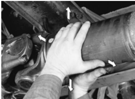
FIGURE 6: CHECK FOR LOOSENESS
