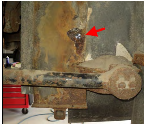
FIGURE 6: CLEANED SPOT ON STRUCTURAL MEMBER
