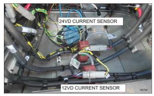
FIGURE 11: 12VD / 24VD CURRENT SENSORS IN MPC (TYPICAL)
