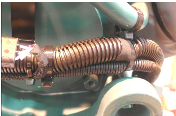
Figure 13: starter cables in a corrugated protective sheath.
