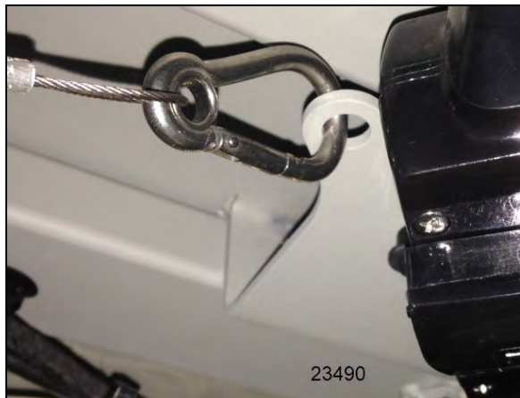
FIGURE 58: PROTECTIVE WIRE INSTALLATION
