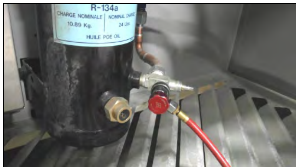
FIGURE 86: RECOVERY UNIT CONNECTED TO RECEIVER SERVICE PORT
