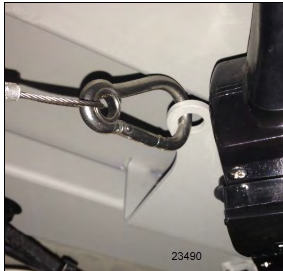
FIGURE 54: PROTECTIVE WIRE INSTALLATION
