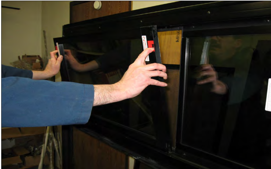
FIGURE 107: REMOVING THE SASH
