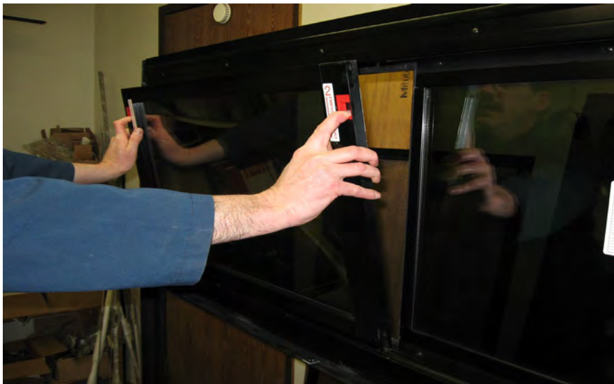
FIGURE 44: REMOVING THE SASH
