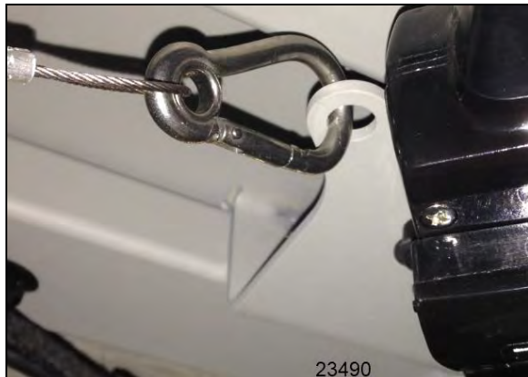
FIGURE 56: PROTECTIVE WIRE INSTALLATION
