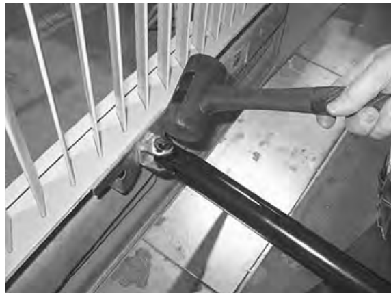
FIGURE 65: DOOR LATERAL ADJUSTMENT
