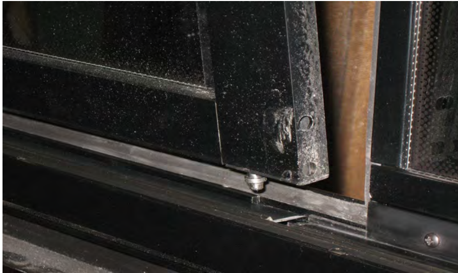
FIGURE 45: DISENGAGING THE BOTTOM OF THE SASH
