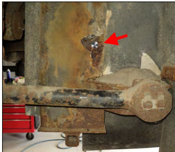
FIGURE 6: CLEANED SPOT ON STRUCTURAL MEMBER
