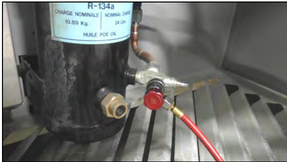
FIGURE 59: RECOVERY UNIT CONNECTED TO RECEIVER SERVICE PORT
