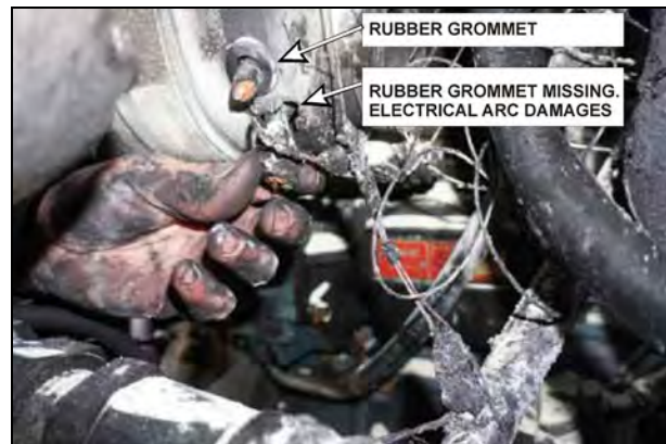
Figure 25: Fire in engine compartment caused by rubbing of power cable against metal edge of Bosch T1 alternator rear cover. Lower rubber grommet was missing when fire occurred. Evidence of electrical arc can be seen.
