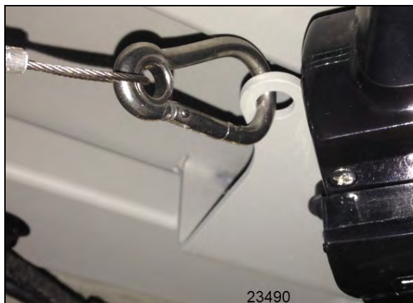
FIGURE 23: PROTECTIVE WIRE INSTALLATION
