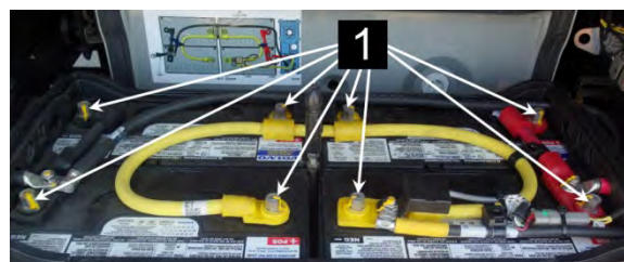
FIGURE 42: INSTALL THE BATTERY CABLE LUGS
