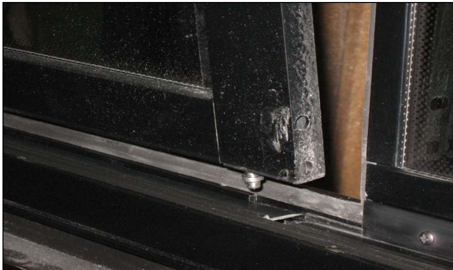
FIGURE 101: DISENGAGING THE BOTTOM OF THE SASH
