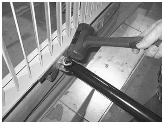
FIGURE 64: DOOR LATERAL ADJUSTMENT
