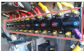
FIGURE 21: MAIN CIRCUIT BREAKERS IN MPC
