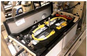
FIGURE 43: BATTERY BANK COVER REMOVED
