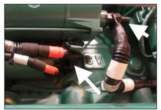
Figure 30: Starter power cable and ground cable lugs protected with Color Guard rubber coating.
