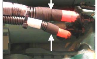
Figure 14: Two layers of fabric tape applied every 3 to 6 inches to prevent the cable from coming out of the corrugated protective sheath.
