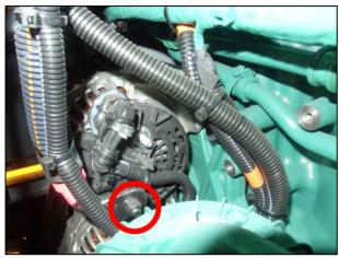
Figure 23: Make sure power cables/positive cables (+) are properly connected to alternator, that stud terminal nuts are properly tightened.
