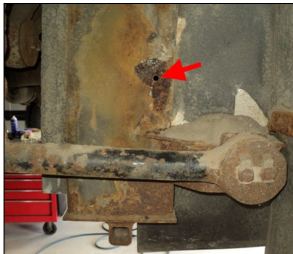
FIGURE 7: HOLE DRILLED IN STRUCTURAL MEMBER
