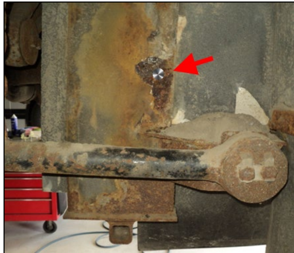
FIGURE 6: CLEANED SPOT ON STRUCTURAL MEMBER
