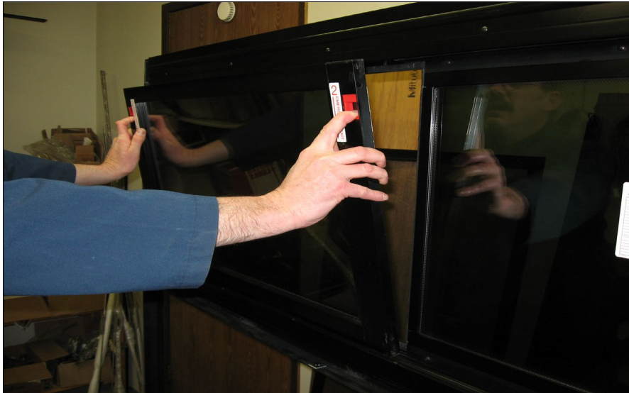
FIGURE 107: REMOVING THE SASH
