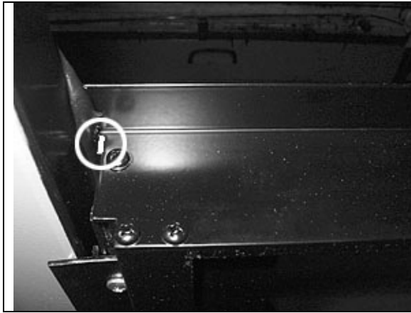
FIGURE 74 : AWNING WINDOW – SEAL THE CHINK
