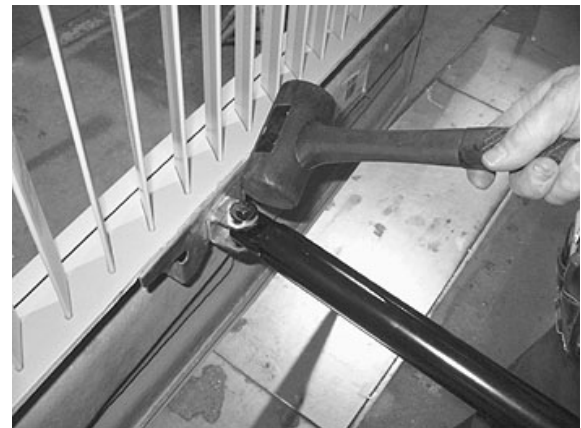
FIGURE 65: DOOR LATERAL ADJUSTMENT
