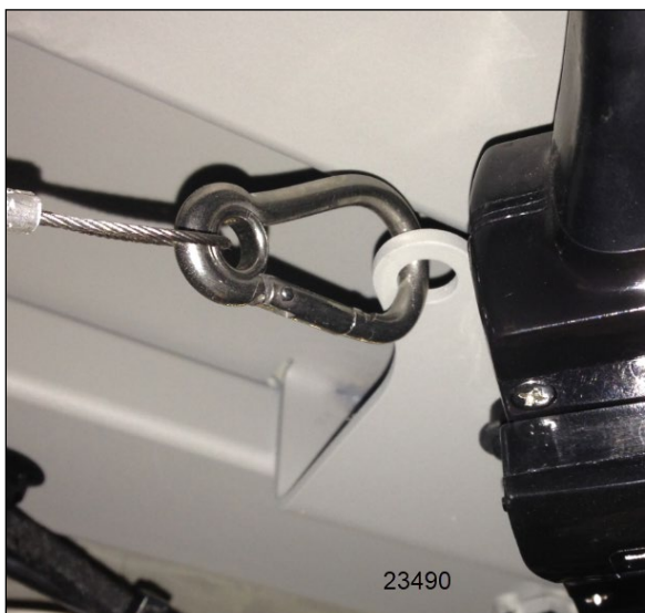
FIGURE 10: PROTECTIVE WIRE INSTALLATION
