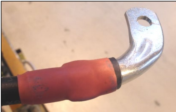
Figure 17: Power cable shouldn't be bent just next to the cable lug. Angled cable lugs are used to avoid mechanical stress.
