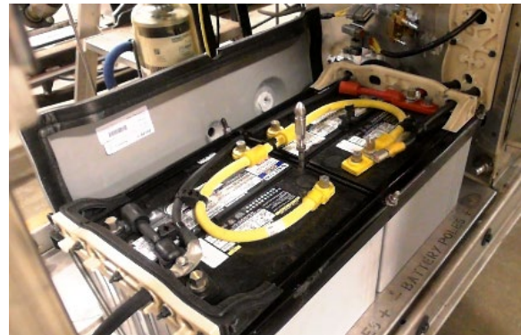
FIGURE 47: BATTERY BANK COVER REMOVED
