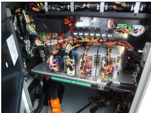
FIGURE 27: FRONT ELECTRICAL & SERVICE COMPARTMENT
