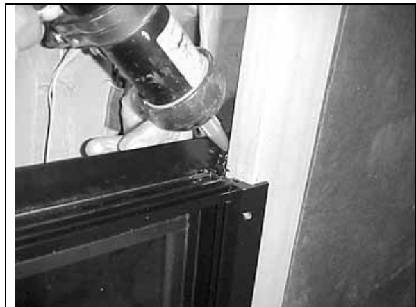
FIGURE 73 : AWNING WINDOW – SEAL THE UPPER CORNERS
