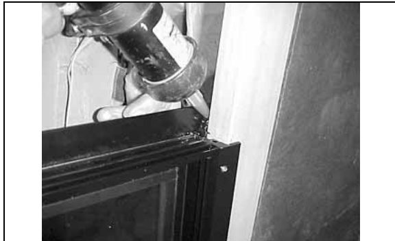
FIGURE 79 : SLIDING WINDOW – SEAL THE UPPER CORNERS
