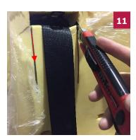
Cut through the foam down the lines with a sharp, (snap bladeretractable) utility knife.
