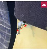
Retract the pull tab through each opening with the pull tab end in a horizontal orientation at the end of the tool.
