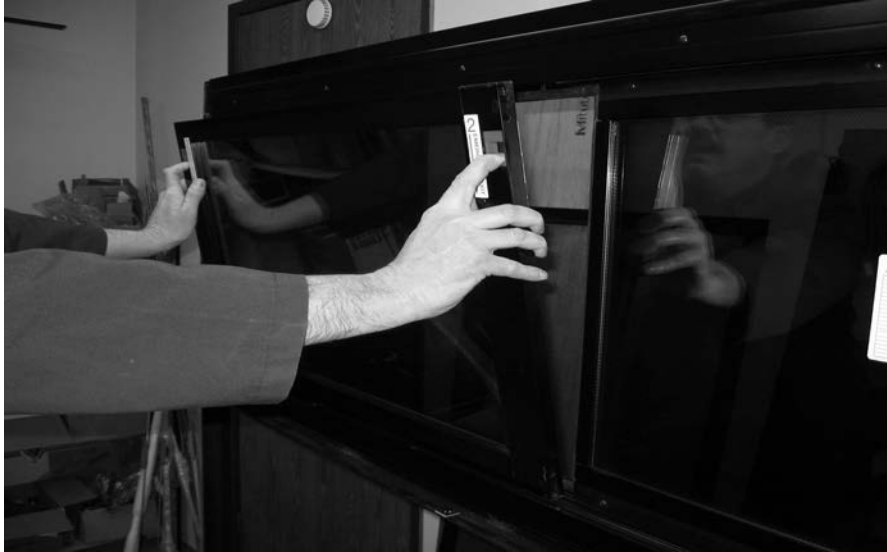
FIGURE 22: REMOVING THE SASH
