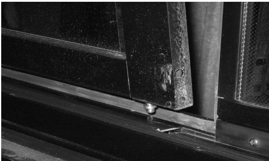
FIGURE 23: DISENGAGING THE BOTTOM OF THE SASH
