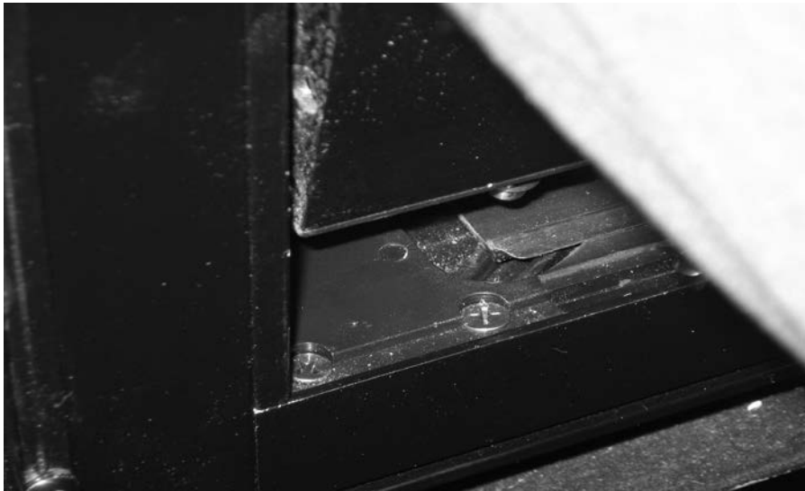
FIGURE 25: POSITIONING THE LOWER LEFT CORNER OF THE SASH
