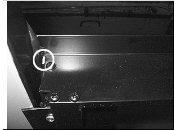
FIGURE 70 : AWNING WINDOW – SEAL THE CHINK
