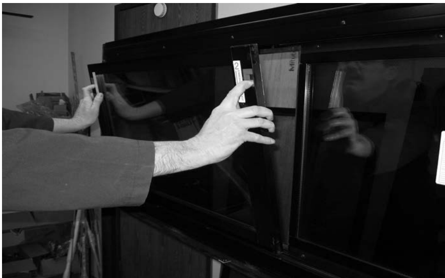
FIGURE 41: REMOVING THE SASH
