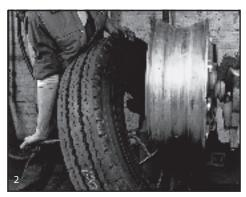
Insert curved end of tool between bead and wheel flange with tool stop against flange. In circular motion, use short successive bites to work the bead over the flange. Push down on tool as bead is worked over flange.
