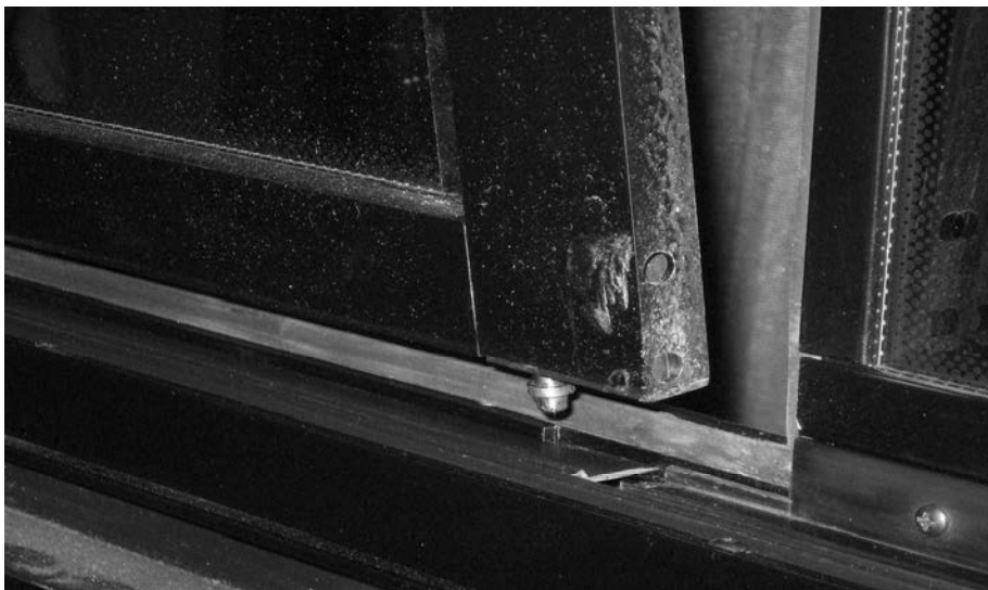
FIGURE 22: DISENGAGING THE BOTTOM OF THE SASH
