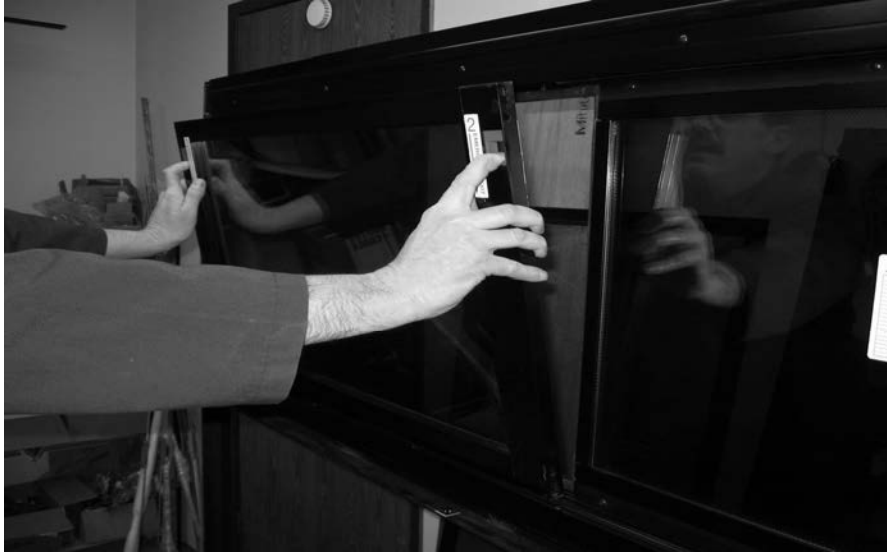
FIGURE 21: REMOVING THE SASH
