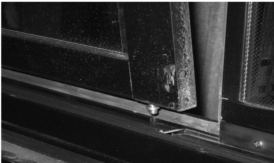
FIGURE 23: DISENGAGING THE BOTTOM OF THE SASH
