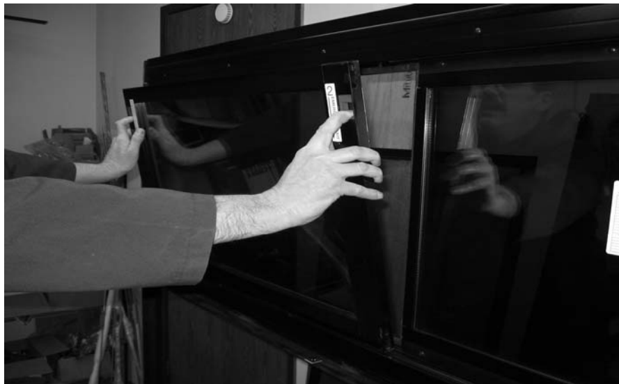
FIGURE 41: REMOVING THE SASH
