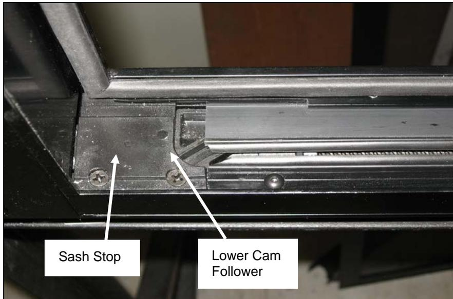
FIGURE 66: PROPER ALIGNMENT
