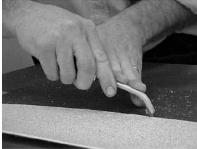
5. Add (about 6 inches) some length to the required length of filler bead to make the joint then cut.
