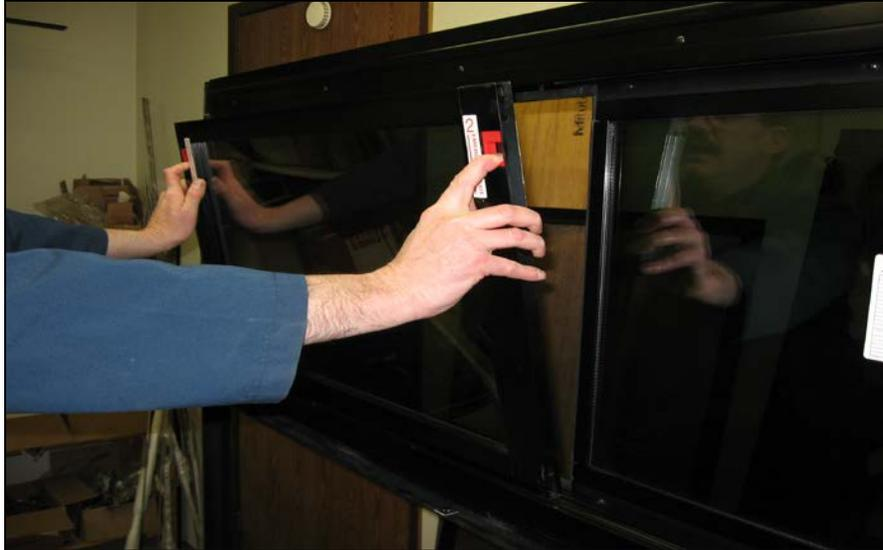
FIGURE 64: REMOVING THE SASH
