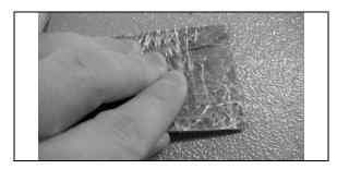
Allow drying for at least **2 hours** then repaint as per paragraph: Minor Repair.
