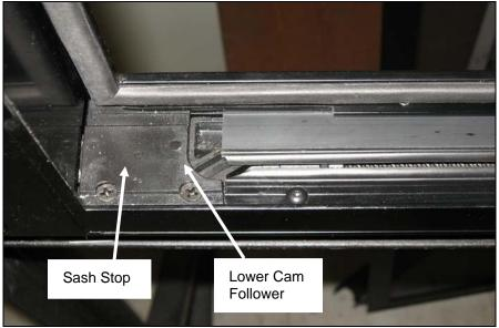
FIGURE 66: PROPER ALIGNMENT
